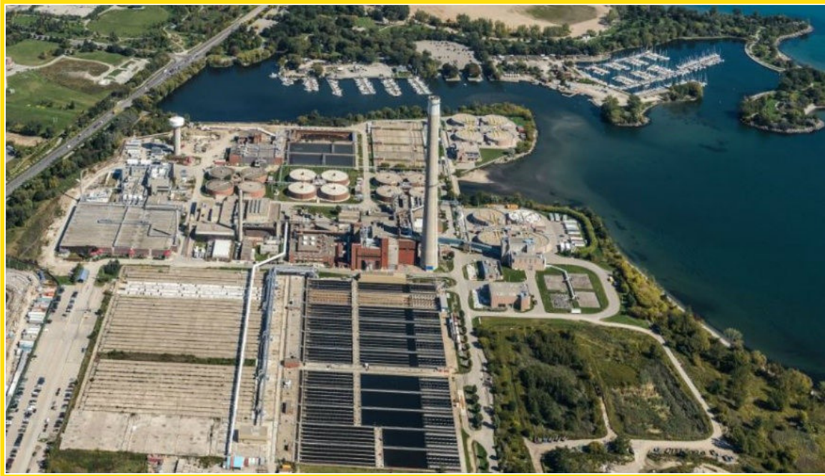
WWTPs with advanced biological treatment can actually transform the levels of PFAS in the influent into other and more numerous forms of PFAS into the air and effluent following biological treatment.
