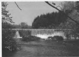
Franklin Dam across the Sheboygan River Alliance of Wisconsin
