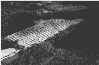
An auto wrecking business in the moraine close to Highway 48, just north of Musselman Lake. A great number of trees were sacrificed to make way for old cars that sit on the sandy soil of the moraine release gasoline, oil, mercury and paint that is absorbed into the sand and travels to nearby streams and ponds.
