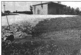
Graffiti-daubed building that shelters Walkerton's well #7
