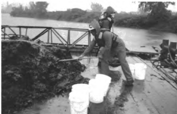
US EPA workers shovel contaminated sediments dredged from Buffalo River for demonstration project in ARCS Program.
